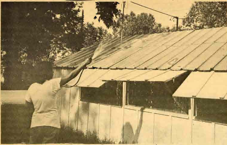
HOME COOLING SYSTEM - You can't live in the Linnell shacks during the day. The temperature reaches 130 degrees inside. Photo by George Ballis.
